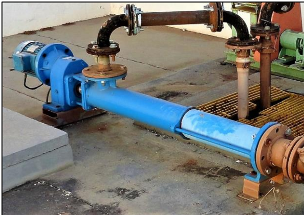
Pumping of sewage
